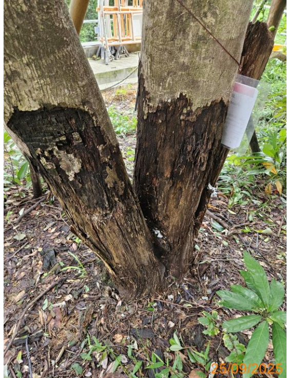
14: U041_Wood damage at trunk union#2
